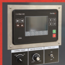
Parallelling Control Panel
