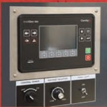
Parallelling Control Panel
